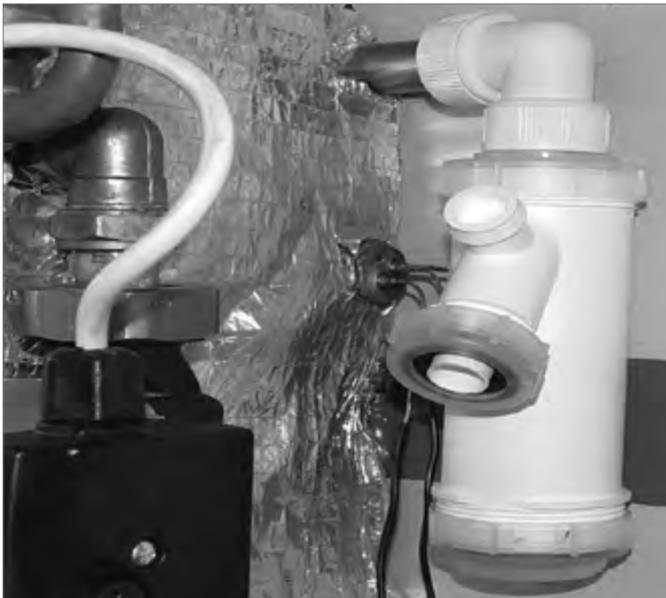
Figure 6-2: Condensate trap
