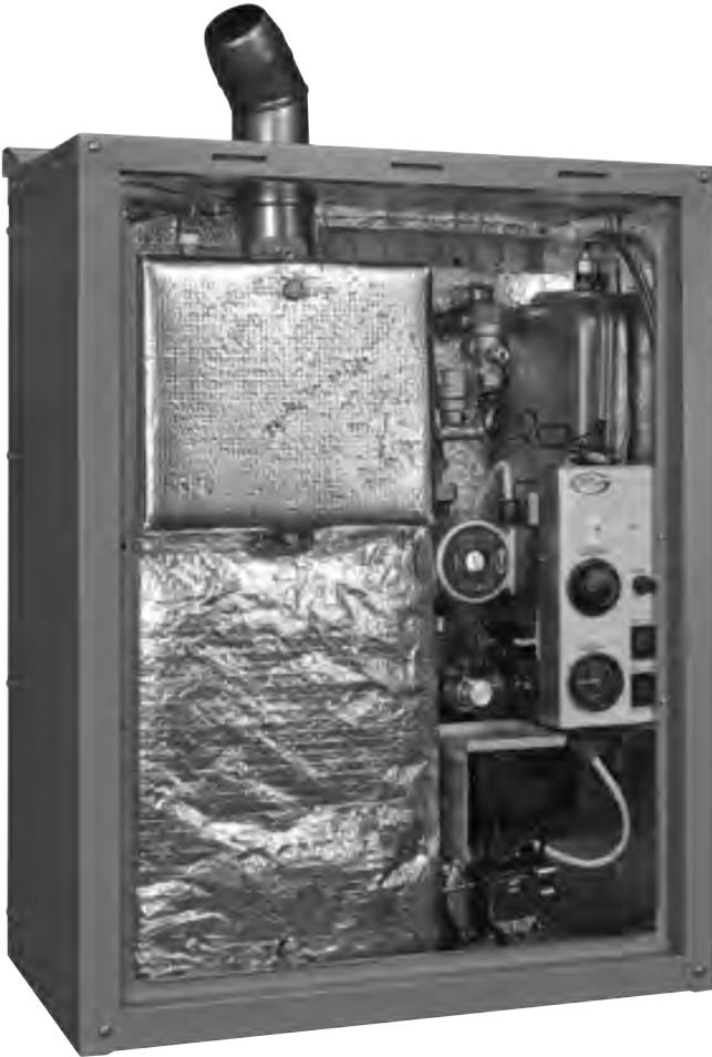
Figure 10-1: Boiler with front panel removed
