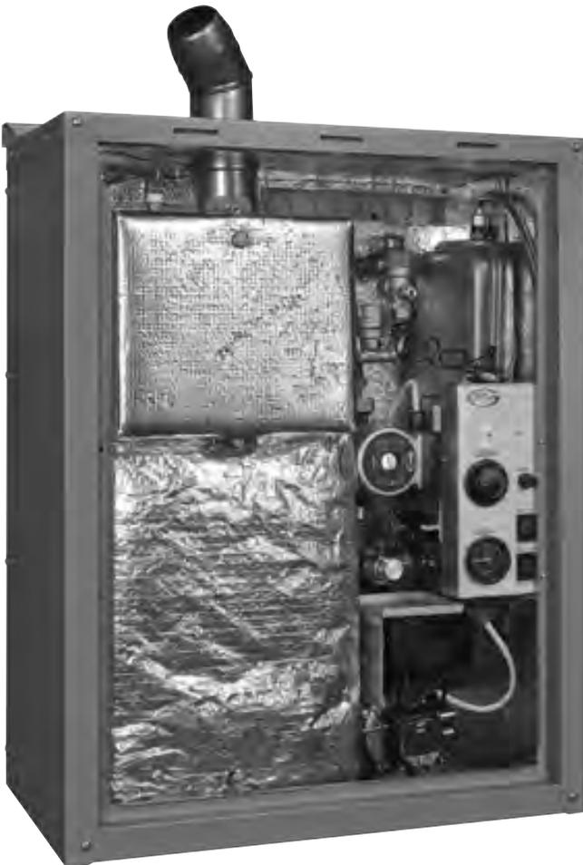
Figure 1-1: Boiler with front panel removed
