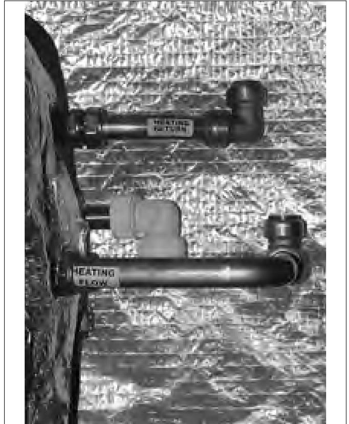
Figure 5-1: Non system boiler flow and return connections
