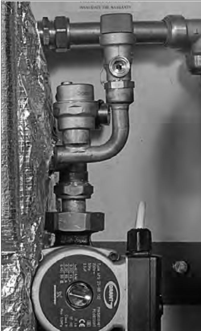
**Figure 4-2:** Removing flow and return pipe
