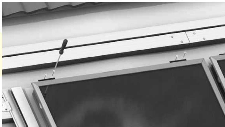
Figure 71: Fixing of the Top Brackets
