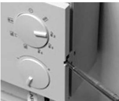
Carefully prise controller out from wiring base
